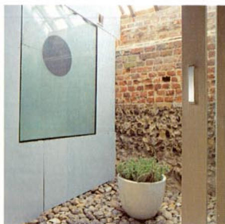
Top: bathrooms in Quaker Barn receive indirect light from internal glazed walls. Above: Quaker Barn's internal courtyard has a cobbled floor and exposed brick wall with flint base. It is roofed with glazed pantiles.
