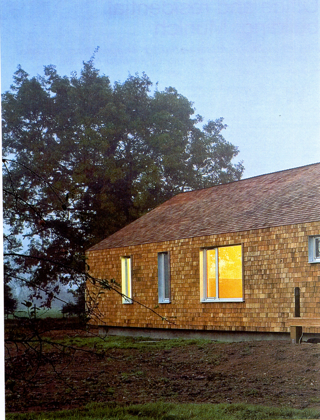
↑ Protruding steel frames articulate the window openings.
