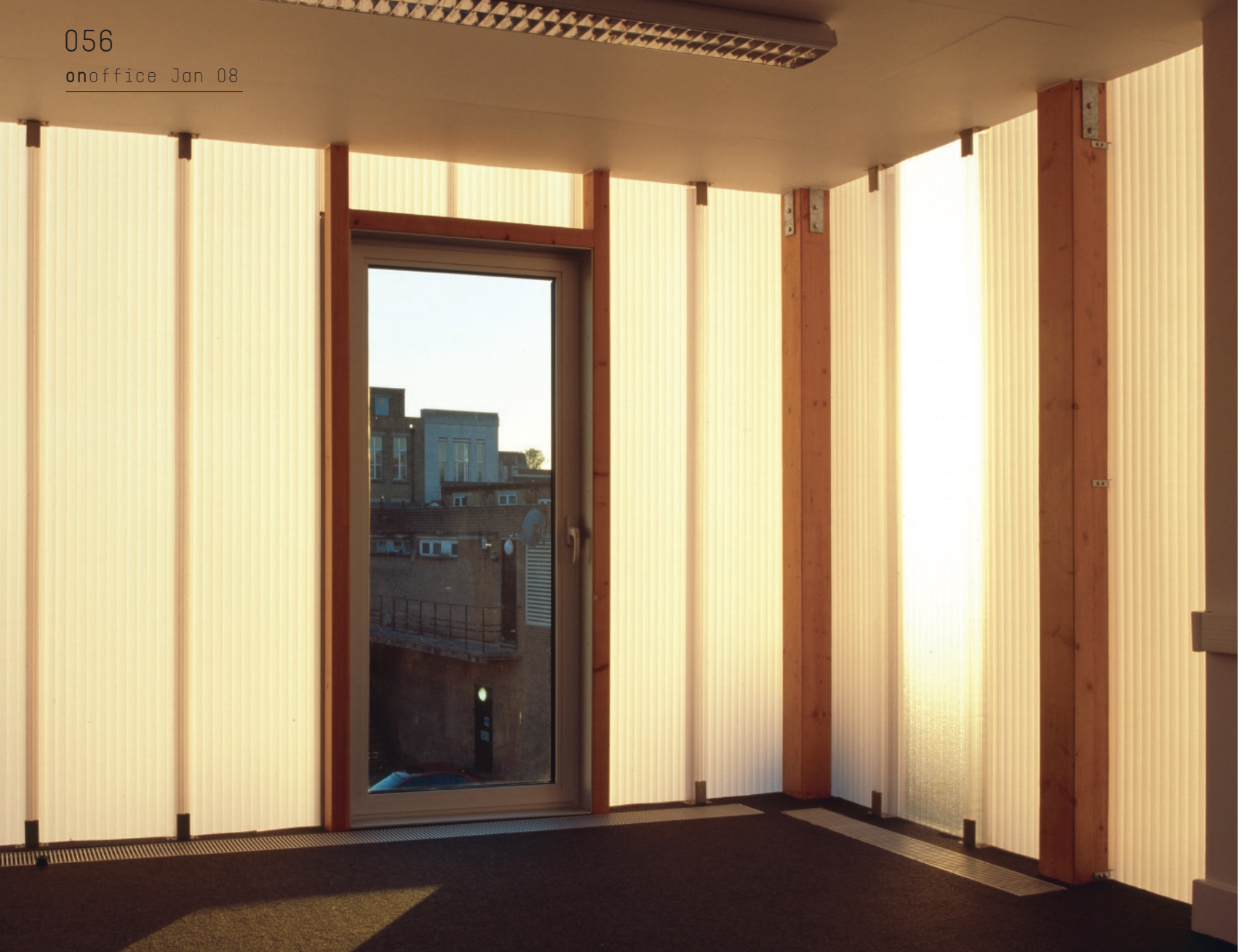
This picture: Translucent polycarbonate walls allow daylight to flood into the building
