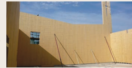
Erection of the panel system, with the tower to the right.
