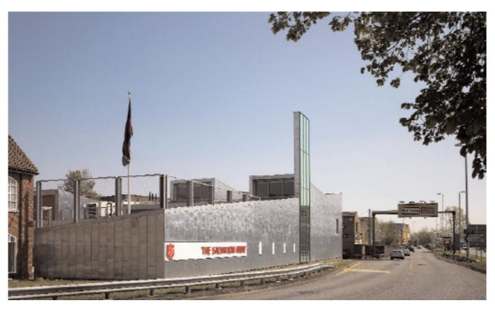
The pièce de résistance of the composition has to be the tower facing Parkway which forces its way up from the zinc cladding of the ziggurat elevation to show off a vertical plane of special film-coated glass, which appears to change colour according to the light and viewpoint. The cut-out silhouette of the cross is evanescent, but just visible through the coloured glass at the top. It is dramatic in terms of strong colour on a prominent elevation, but subtle in terms of visual symbolism.
