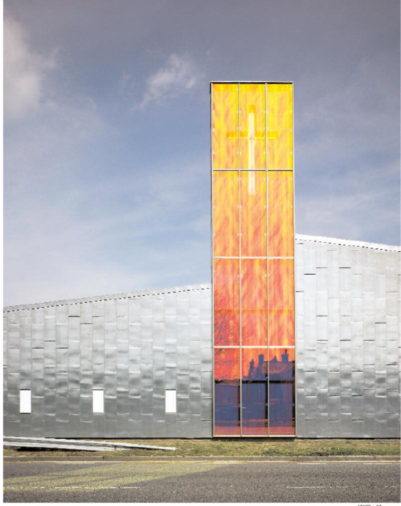
Above The entrance canopy on the north elevation is integral to the solid timber structure. Location plan 1 Baddow Road, 2 Goldlay Road, 3 Parkway. Opposite The 13 metre tall tower, made from the longest cross-laminated timber panel available, is clad in radiant film reflecting a spectrum of colour.
