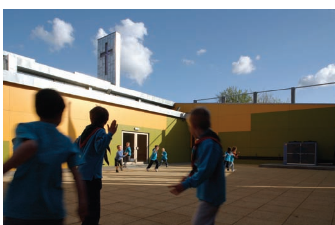
The two principal facades extend to enclose a courtyard.
