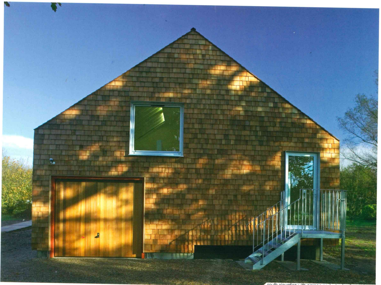
south elevation with garage and raised gallery entrance
