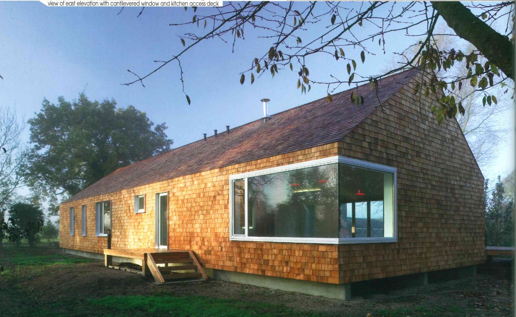
view into the main living area from the west raised access view of east elevation with cantilevered window and kitchen access deck
