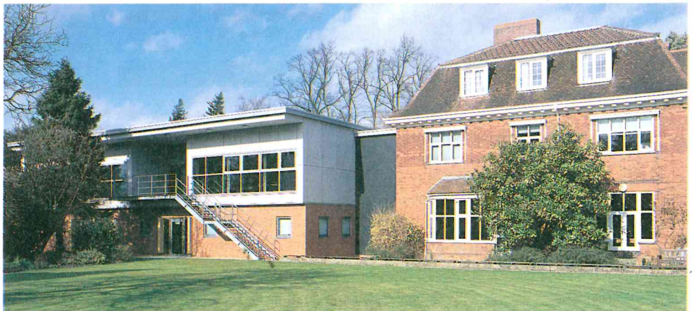
Right The south elevation contrasts the red brick of the ground floor with the rainscreen cladding to the first floor.
