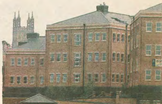
Brick walls: Leeds magistrates' court, top, and Gloucester county and crown court. Photographs by Justin Slee, top, and Adrian Sherratt
