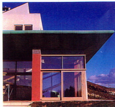
3—When raised, the glazed screens form the front of the house, and give the public areas a panoramic view of the sea
