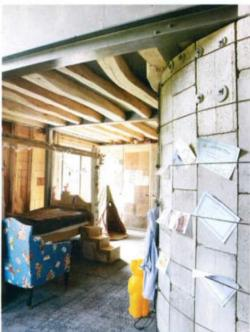
left, above and below Two existing silos, made of concrete blocks, were dismantled and rebuilt, concealing Ben and Freddie's bedroom and en suite on a steel-framed mezzanine, and Wilhelmina's bedroom under it right 'We had to repair a lot of damage to this side of the house,' says Ben, 'which meant the planners were more lenient about the windows here. They did stipulate that they should be Clement Windows, though - favoured for their very thin profile'
