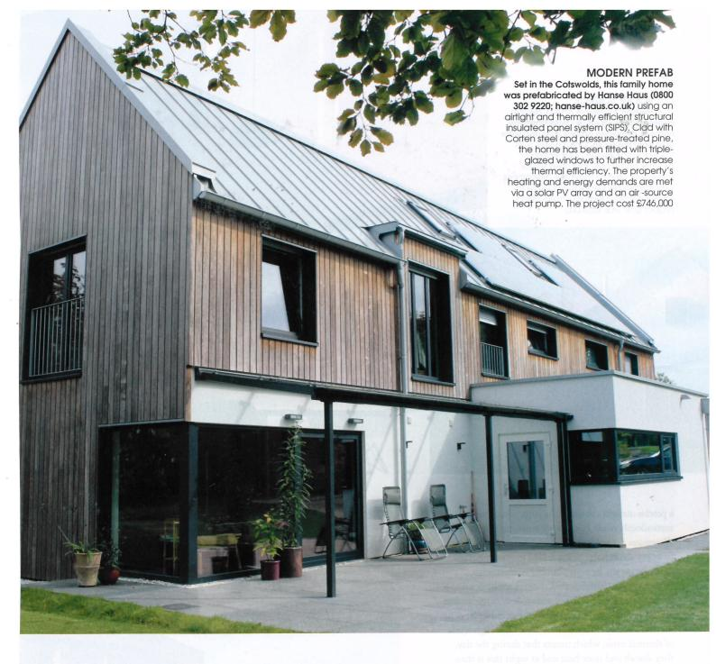
helping you achieve a low-energy lifestyle, you need to go back to basics to ensure your tech add-ons can work at optimum efficiency. Taking a fabric-first approach to the envelope of your home means you are prioritising the design and construction to minimise the need for heating and cooling in the first place.
