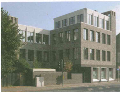
51 Hills Road, Cambridge Gort Scott for private client Contract value: Undisclosed GIA: 780m 2
