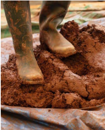
Figure 3. Mixing the structural CobBauge mix by machine or foot. Photo: Plymouth University, CobBauge project (2021) (left), François Streiff (right).
