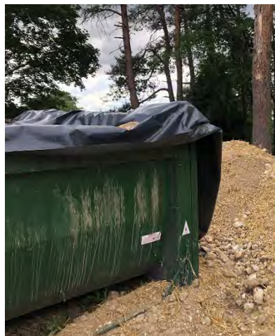
Figure 12. Tarpaulin sheet covering the cob material mix. Photo: Katey Oven.
