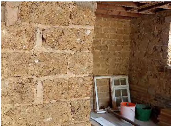
Photo 9. Renovations to an early 20 th century clay lump house at Blo' Norton, Norfolk. The blocks were made from locally-sourced Lowestoft Till mixed with chopped straw. Photograph TD Holt-Wilson.
