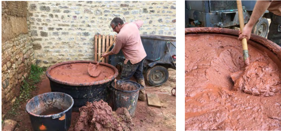
Figure 6. Mixing the subsoil with water, in a large bucket, to form the clay slip. Photo: François Streiff.
