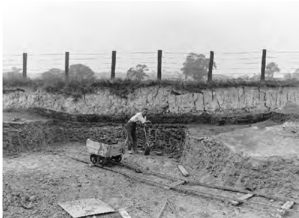
>>> Photo 6. Digging clay from the Lower Coal Measures at Clough Green Pipe Works, Cawthorne, West Yorkshire, 1928. Fireclay is being extracted from beneath a shallow coal seam. Photograph courtesy British Geological Survey P204533.
