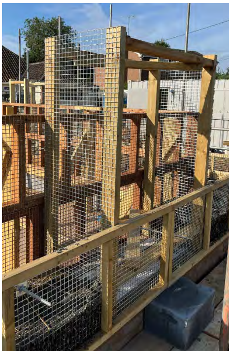
Figure 38 The plywood & mesh window boxing (left), & boxing embedded within the CobBauge construction (right). Photos: Katey Oven (2022).
