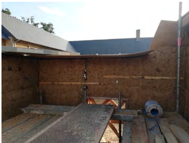
Figure 39. Sheets of timber protecting the tops of the CobBauge wall. Photo: François Streiff.
