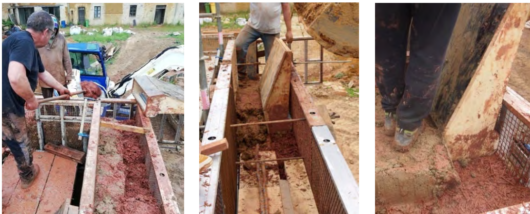
Figure 32. Placement tool being used on site. Photo: François Streiff.
