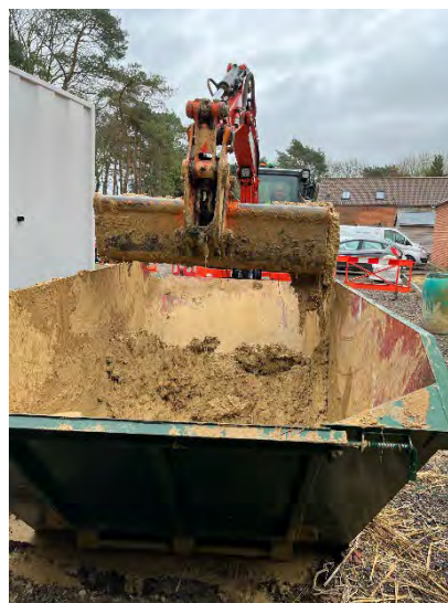
Figure 4. Mixing the structural cob mix in a skip with a digger bucket. Photo: Katey Oven.
