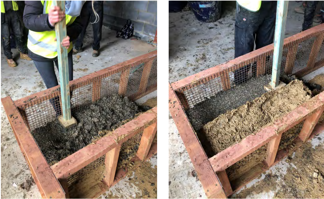
Figure 30. Tamper tool and technique for thermal layer. Photos: Tom Booen.
