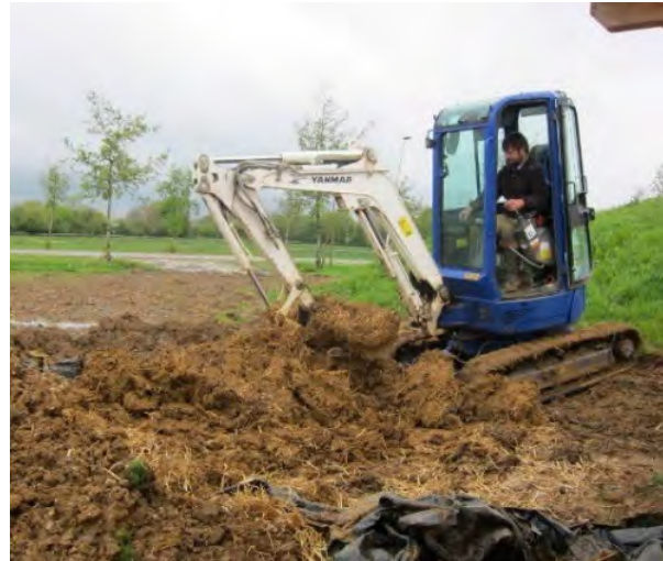
Figure 3. Mixing the structural CobBauge mix by machine or foot. Photo: Plymouth University, CobBauge project (2021) (left), François Streiff (right).
