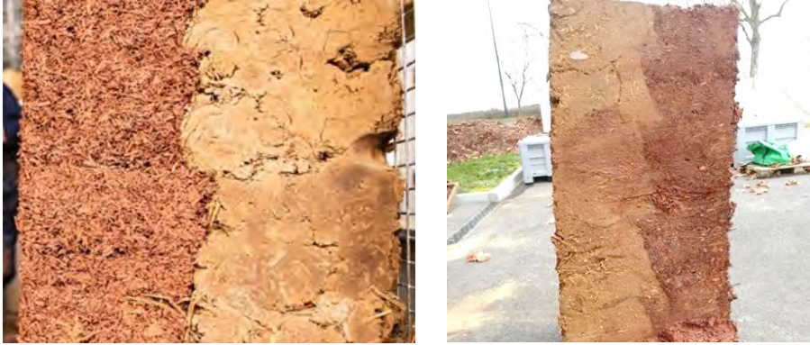
Figure 27. Angled saw toothed joint between thermal and structural layers. Photos: University of Plymouth, CobBauge project
