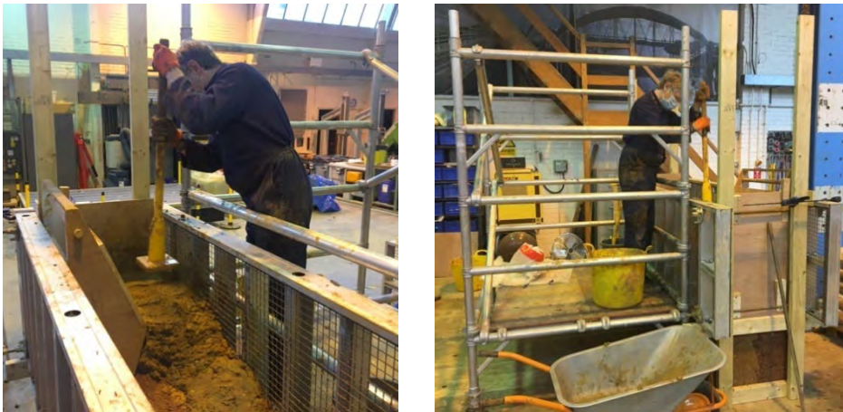
Figure 41. Using a small scaffold platform to aid low level construction.
