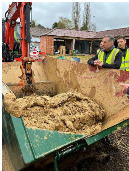
Figure 4. Mixing the structural cob mix in a skip with a digger bucket. Photo: Katey Oven.
